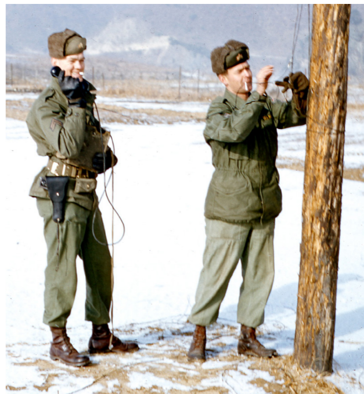
Ray Christensen (left) and Bruner checking telephone lines
