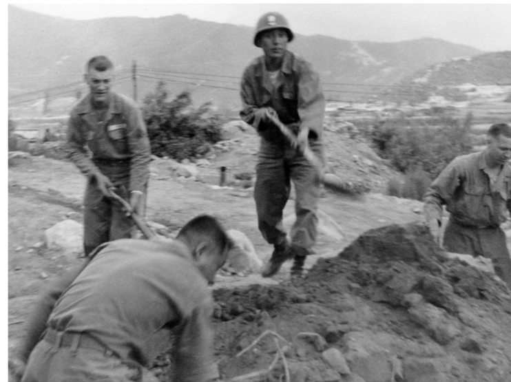
Bob Hansen (right) digging trenches
