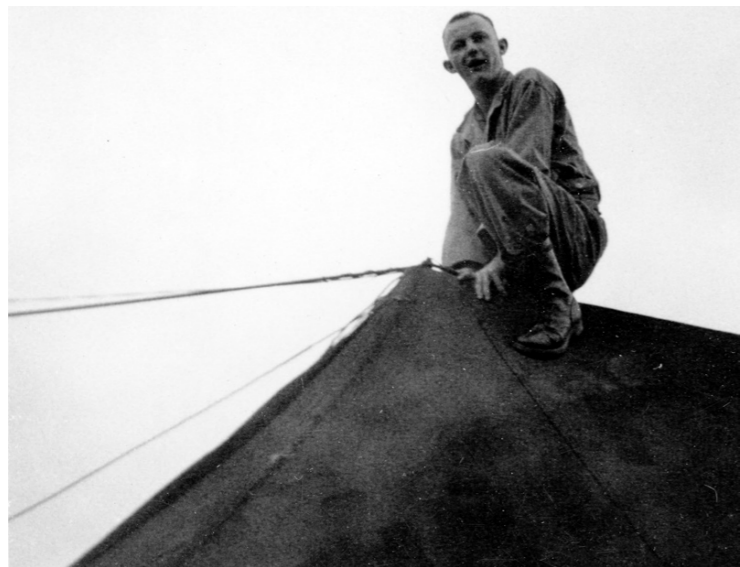
Whitford putting in a communication wire.
