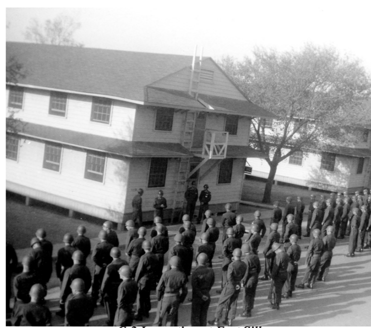
C-2 Inspection at Fort Sill
