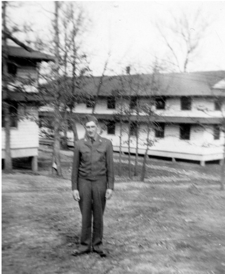
Two story wooden barracks at the Engineering section where Herb Eich (shown above) lived on the Rhine base at Kaiserslautern.
