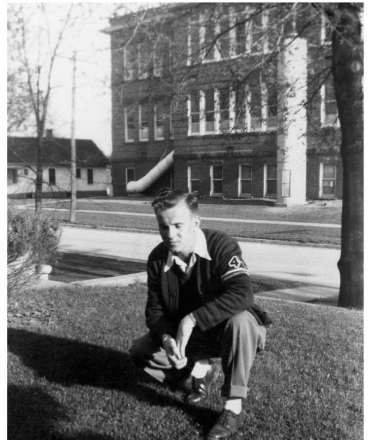
Charles Schumann on the north side of First Street. The old grade school to the south. Note the spiral fire escape along the north wall.
