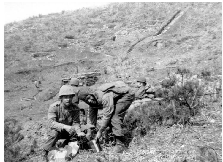
In the background is a trail to the front line. Note the chimney on top of the bunker. This was a sleeping bunker.
