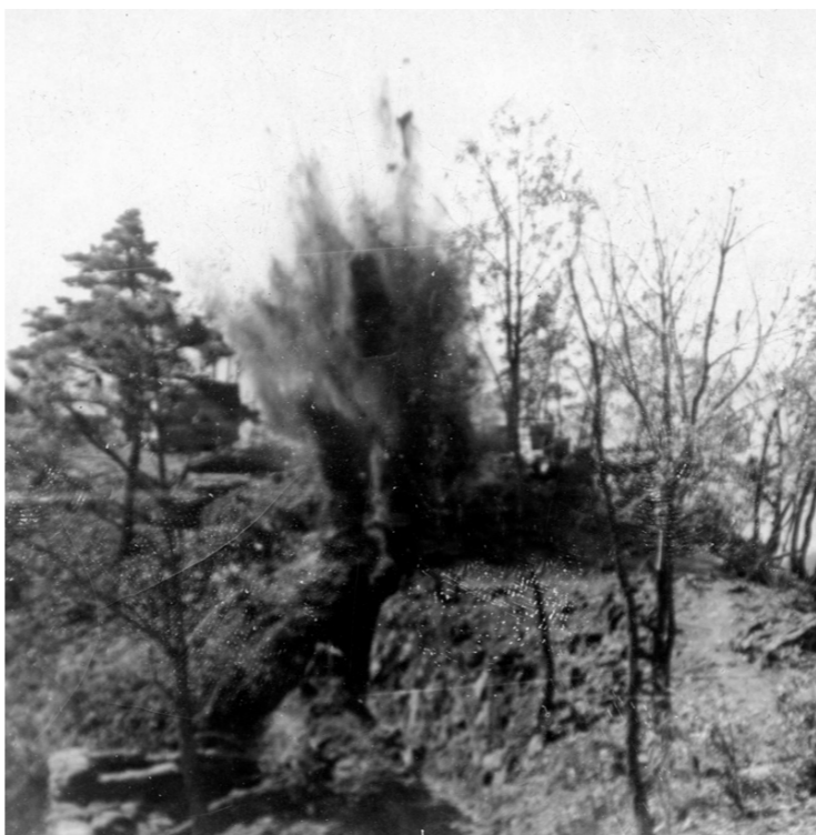
November 1953 Blasting a bolder in the trench. They took the picture from behind a tree and still almost got clobbered by a rock. Explosives Engineers would come in and do the blasting and then Dan and the other men in the company would clean up the debris in the trenches.
