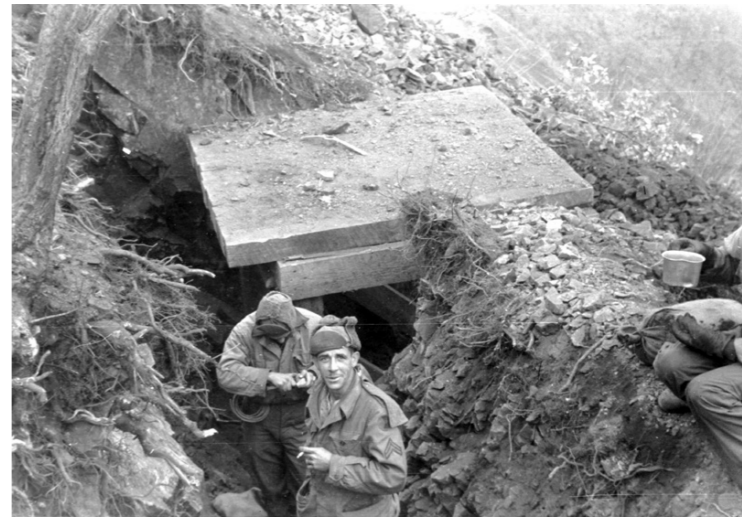
Setting a charge in the trench on the hill for the new defense line built after the war. Korean civilians were hired to carry these 8x8 timbers up the hill to this location. These timbers formed the roof of the bunker before sand bags were placed on top.
