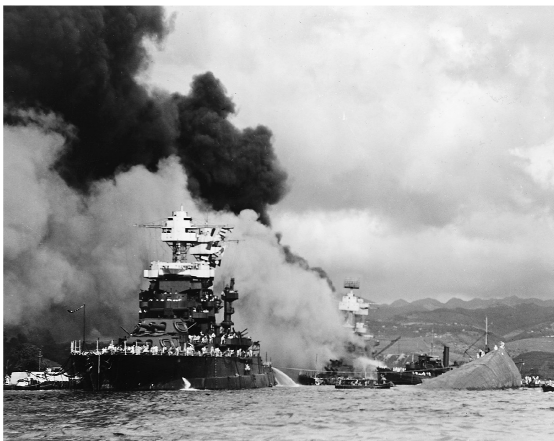
The Maryland on the left, with the capsized Oklahoma on the right, while the West Virginia burns in the background.
