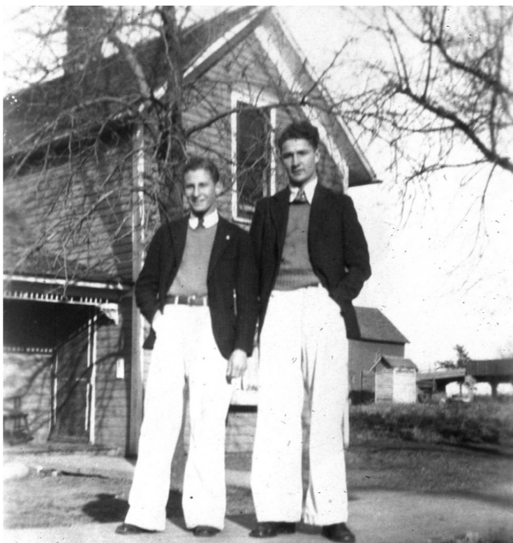
Franklin Vollmer & Don Owen - you can see the old East Street bridge over the Milwaukee RR tracks in the back right.
